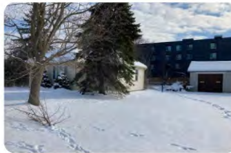
Subject Site, 426 Niagara Drive, Oshawa
