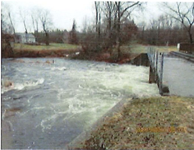
Photo 55 Downstream View of Bennett Dam
