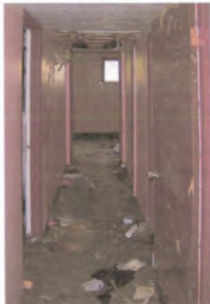
Finished basements experience far greater damages than unfinished basements when the basement floods.
