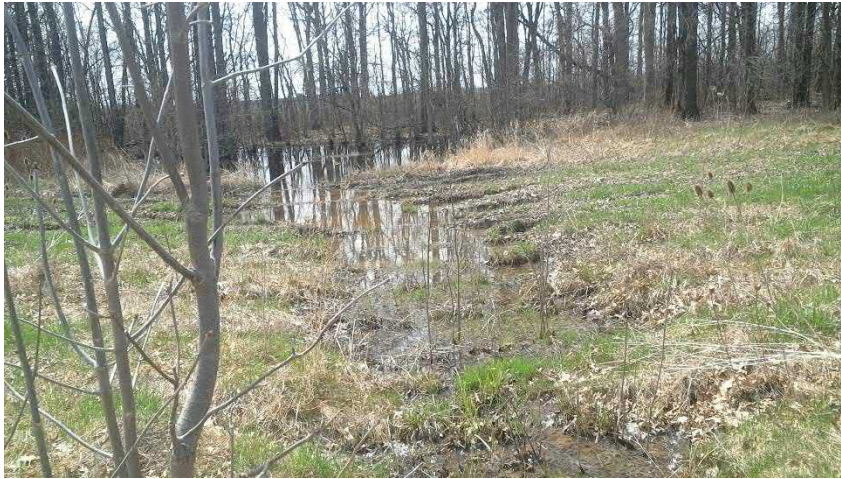
Photo 9. One of the many constructed drainage features actively draining the Slough Forests (30 April 2019).
