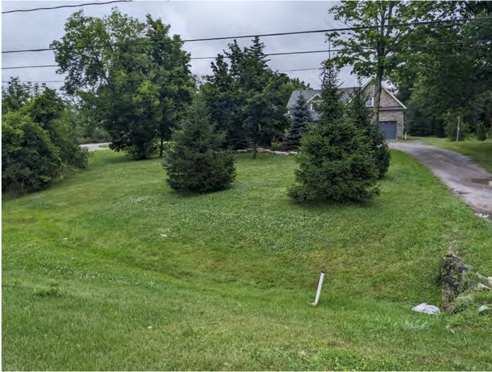
Photo 2 – Front perspective of 424 Aqueduct Street (Part of Subject Lands – House to be demolished)
