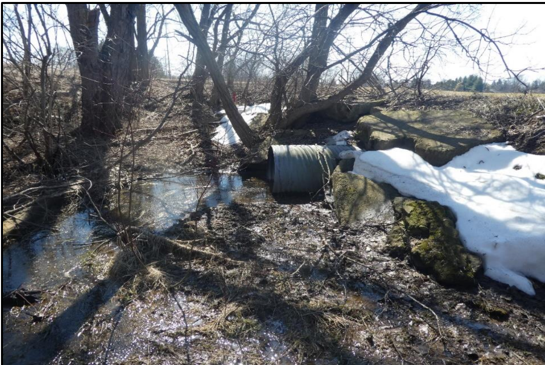
Photograph 9. Soccer Field 170 Piped Section Outfall to the Channel of the Drain in March
