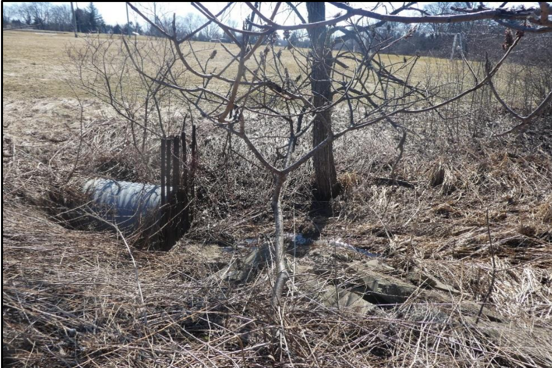
Photograph 8. Stormwater Pond Outfall Culvert in March
