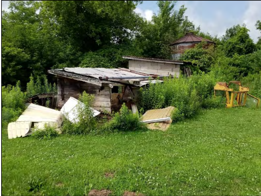
Image 9: View of old derelict farm buildings.
