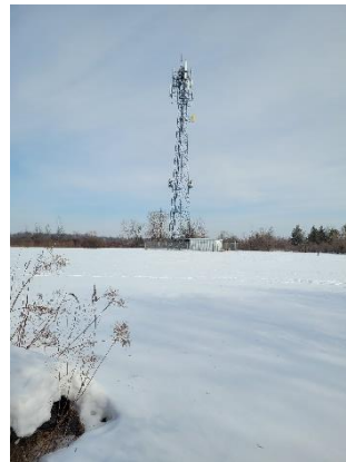
Picture 22: View of the bell tower located on Site, towards the southern portion of the site, facing east.
