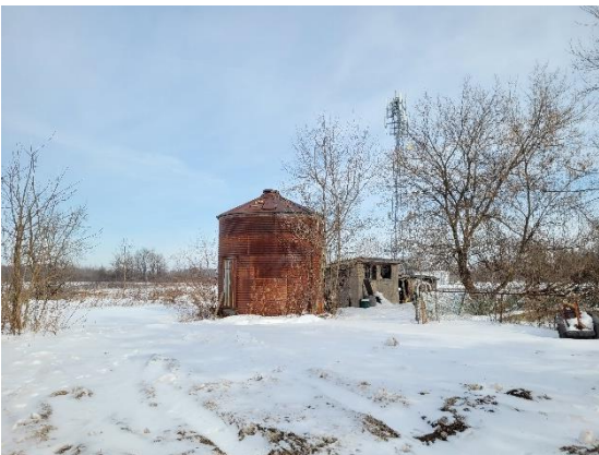
Picture 21: View of the silo to the north of Site Building A, facing north.
