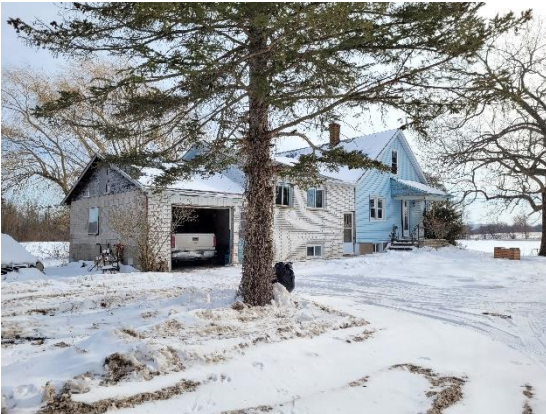
Picture 13: View of Site Building A, facing southeast.
