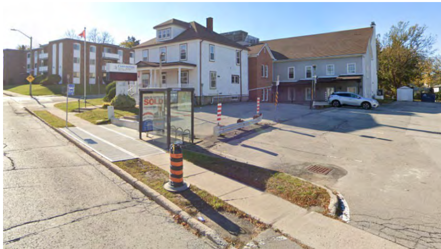
Existing: 5925 Summer Street, Niagara Falls (2020)
